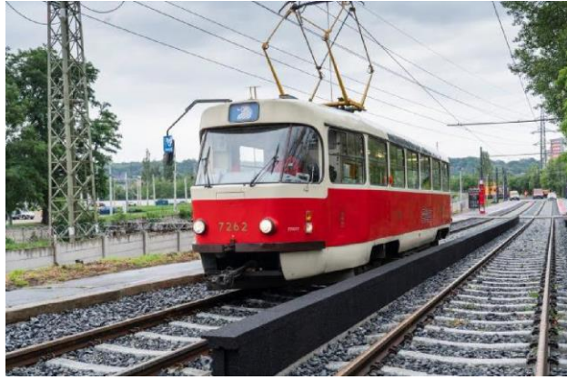
Figure 4: Example of low-height barriers installed in Prague.
