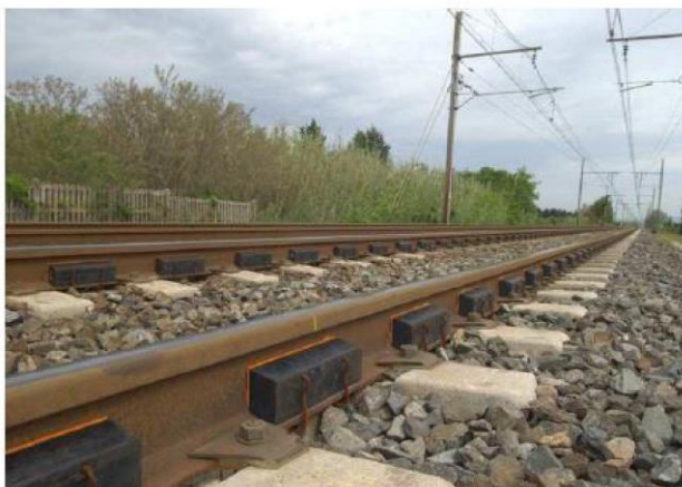
Figure 9: Absorbers tested on a railway by Vossloh company [16].
