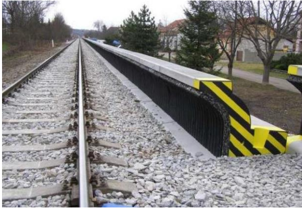
Figure 11: Circular profile used in Czech Republic (interhecplus.cz) for a railway solution.
